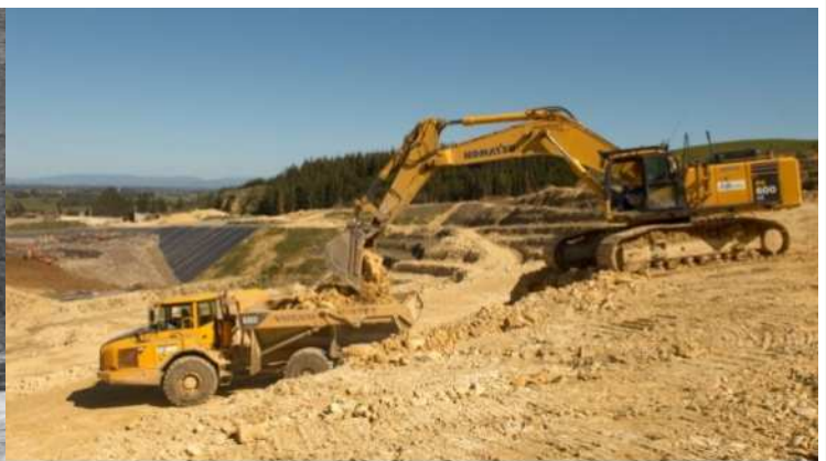
The power of modern equipment means rock is ripped from the ground using a 60 tonne excavator.
